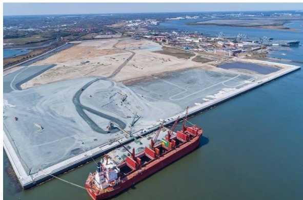
3 Port, Project, and Logistics Services
